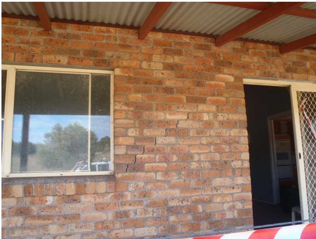
Photo 2: Damaged brick work “Barton Hedge”
